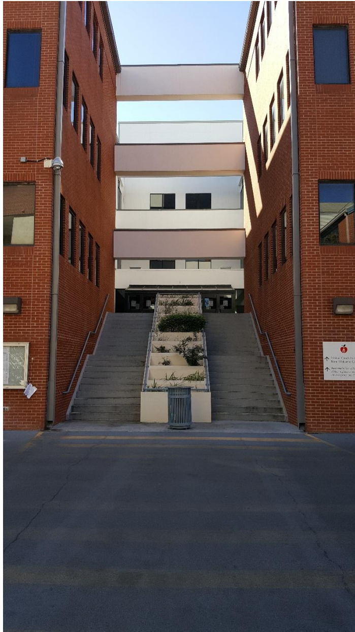
Carruth Administration Center (CAC), 1111 West 6 th Street
