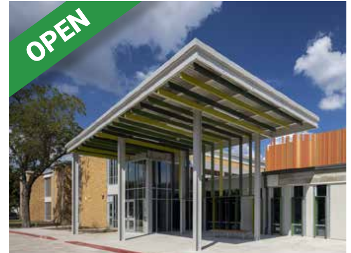
Sánchez Elementary School Main Entry
