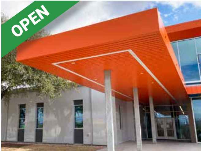
Norman-Sims Elementary School Main Entry
