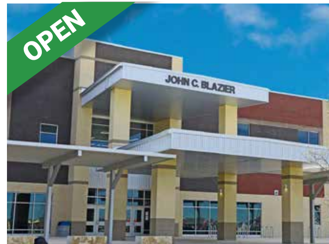
Blazier Elementary School Intermediate Site main entry
