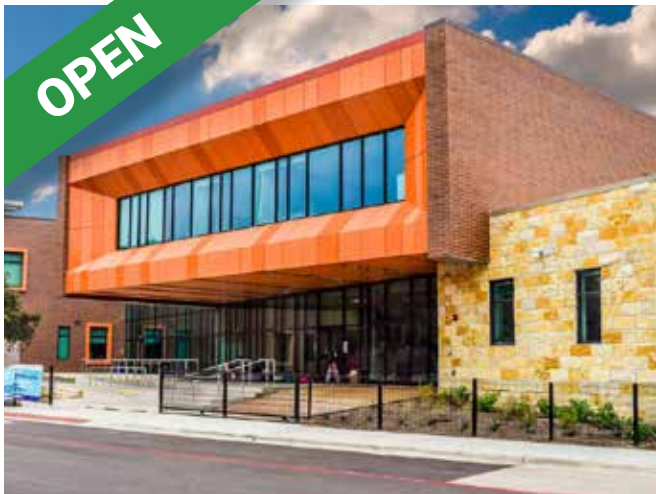
Doss Elementary School Main Entry
