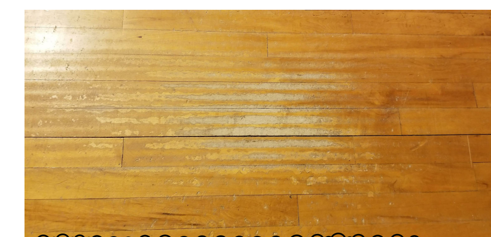
PHOTO 3: SAND FLOORING DOWN TO THE WOOD.
