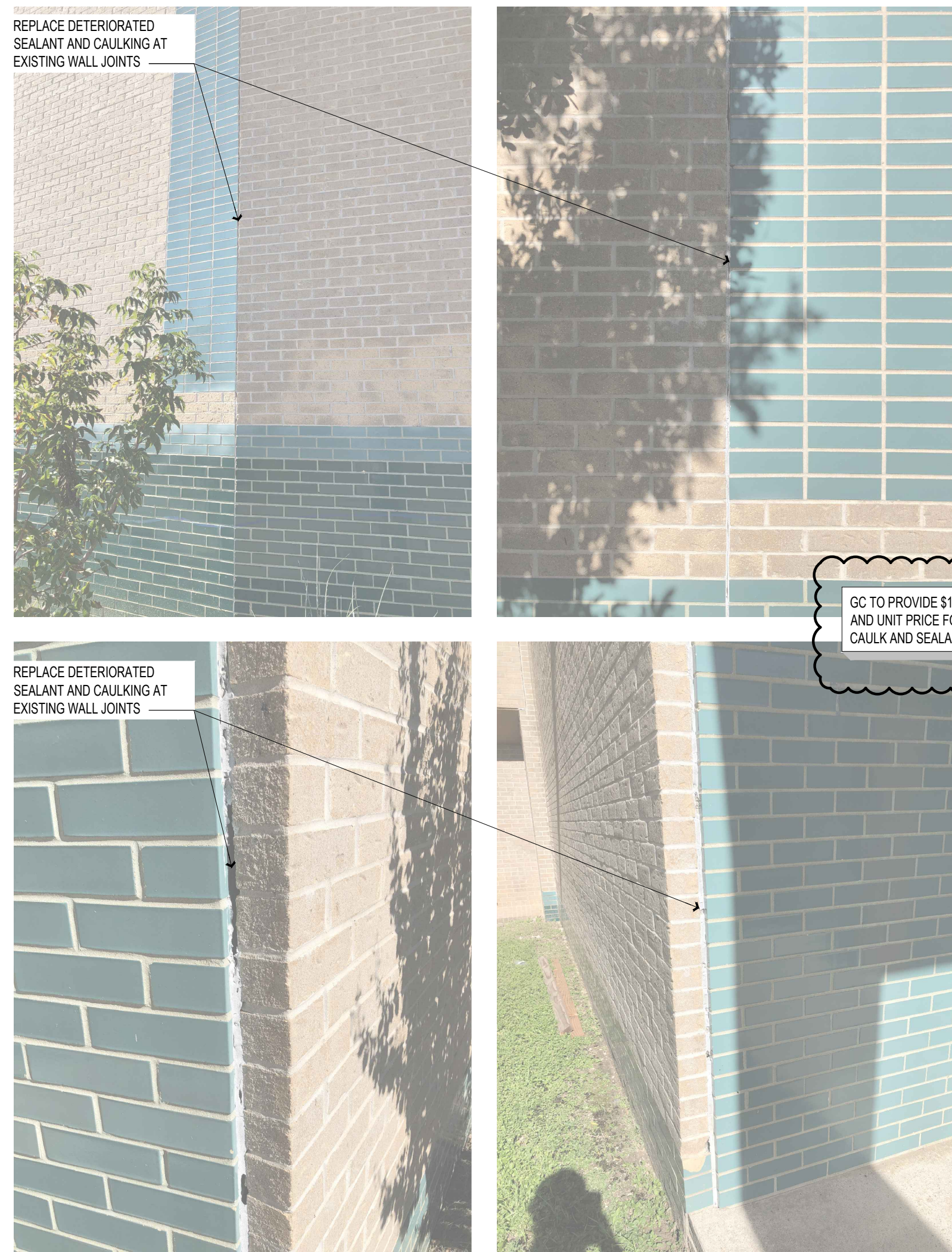
4 EXTERIOR WALL JOINTS SCALE: NTS
