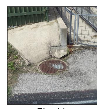
Plumbing Corroded Drain
