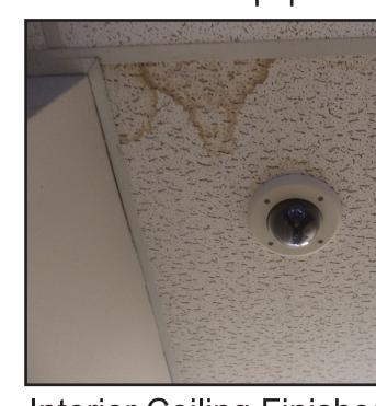
Interior Ceiling Finishes Damaged & Stained Tile
