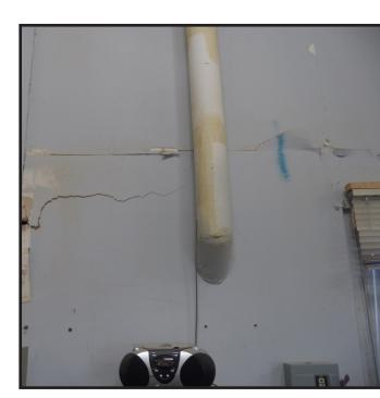
Interior Wall Large Cracks
