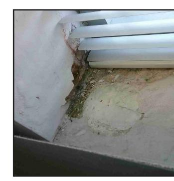
Interior Windows Corroded Frame
