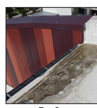
Roofing Ponding, Water Damage
