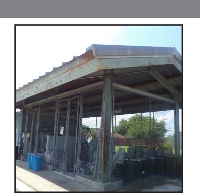
Exterior Walls Rusted & Corroded
