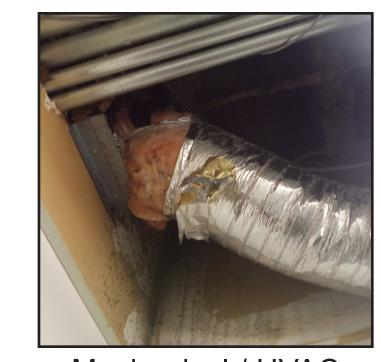
Mechanical / HVAC Damaged Insulation
