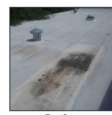
Roofing Water Ponding
