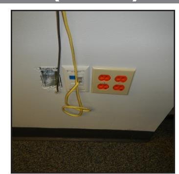
Electrical Distribution Exposed Wires
