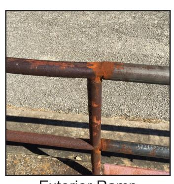
**Exterior Ramp** Rusted Hand Rails
