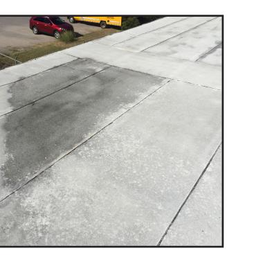
Roofing Water Ponding Damage
