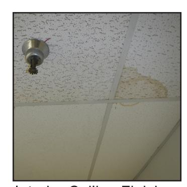
Interior Ceiling Finishes Stained & Damaged
