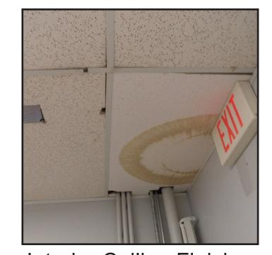
Interior Ceiling Finishes Water Damaged Tiles
