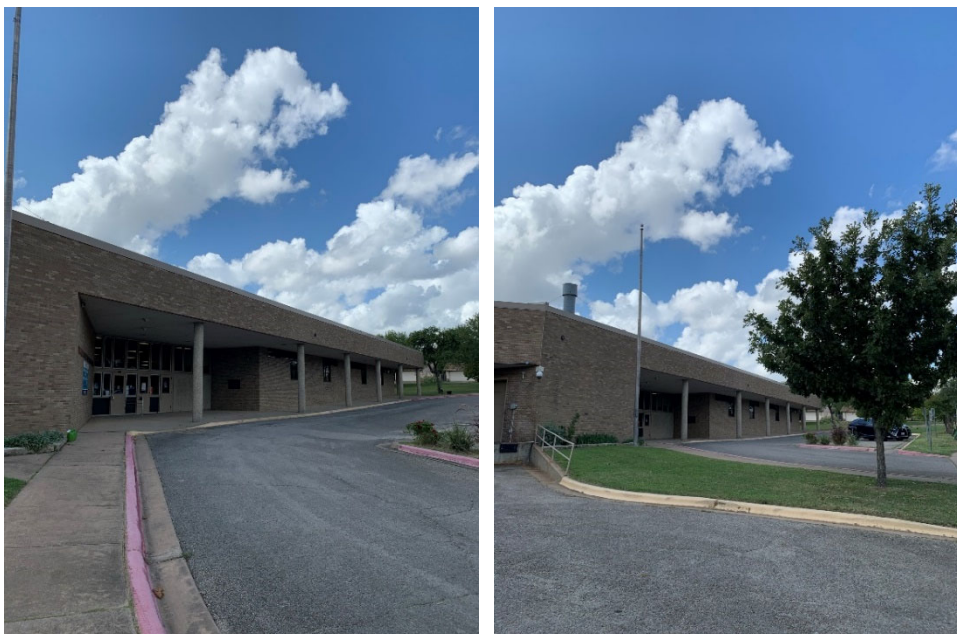
Minimal parking in front for visitors and short stack space. Signage is inadequate.
