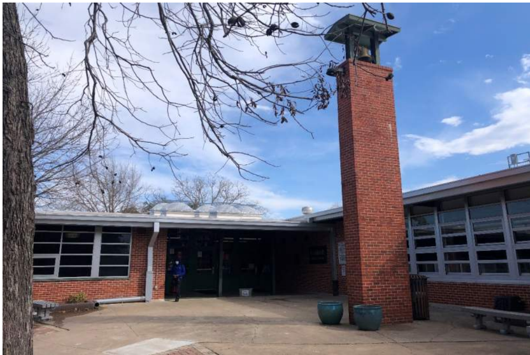
School Entry: Not very inviting or open. Belltower adjacent to entry is well-loved and is one aspect of the campus that should not change in the future.
