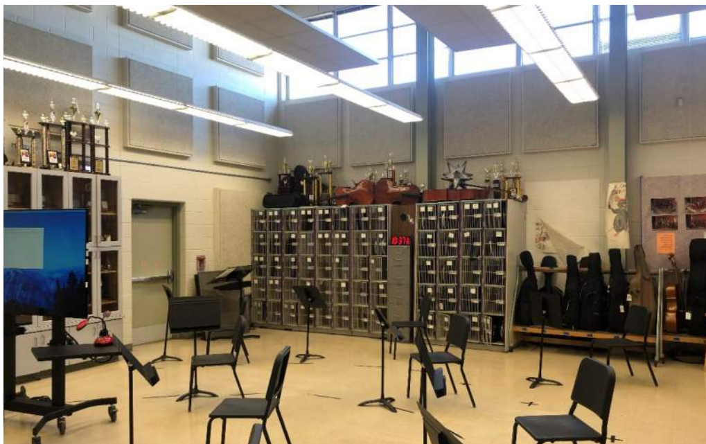
Orchestra Room: Undersized per Ed Spec and missing support spaces. Overall, the room is in satisfactory shape but cannot accommodate growing program.
