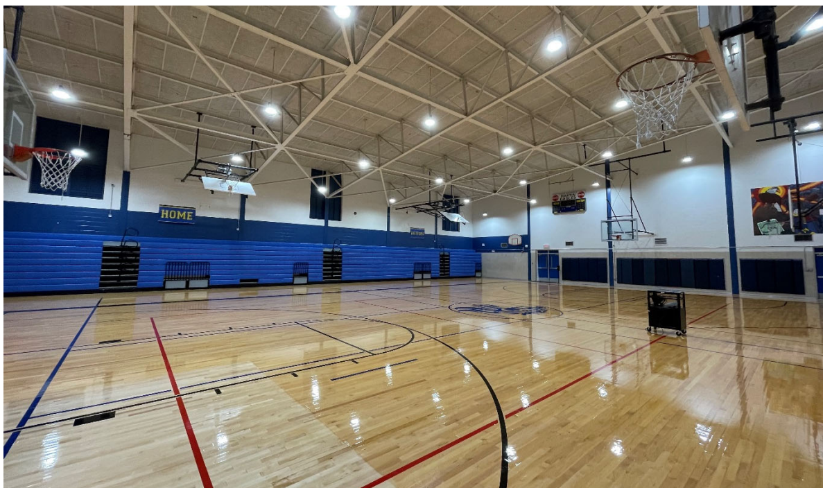
Large and small gym are appropriately sized and in good condition. Patch of new flooring can be seen in the foreground of the photo.
