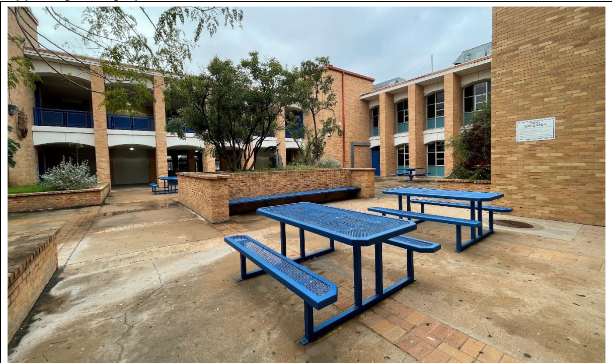
Courtyard spaces are equipped with furniture but lack shade canopies or power access.
