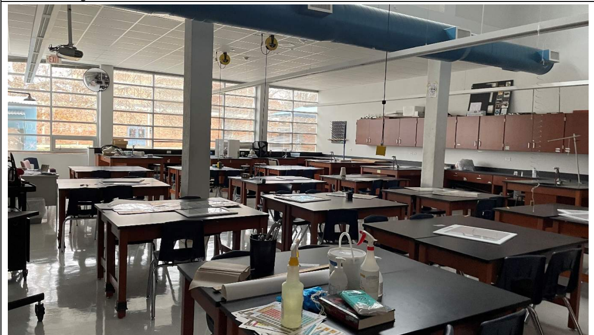
Science Lab Renovation: Adequate space, storage and prep area.
