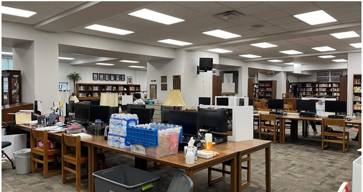
Media Center: Library in good condition, but most furniture is not reconfigurable or easily movable. No breakout rooms or individual study spaces.
