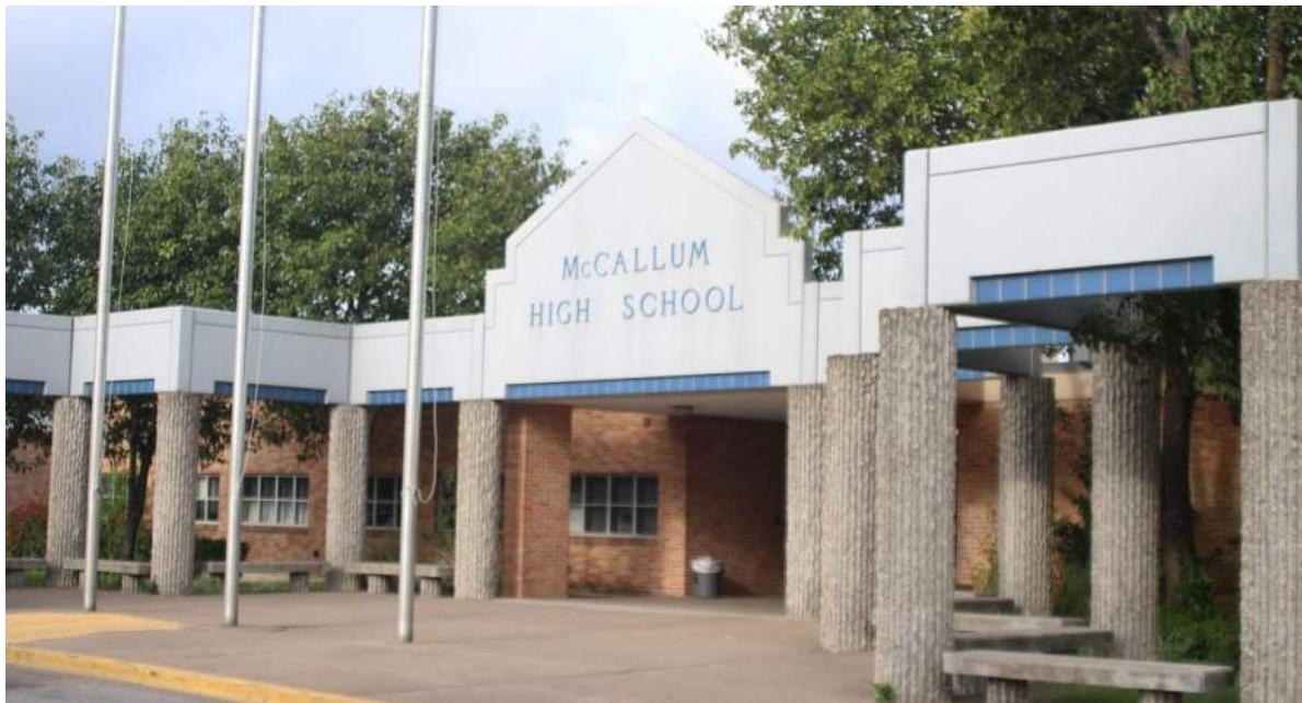
Exterior of school is dated, but in good condition.
