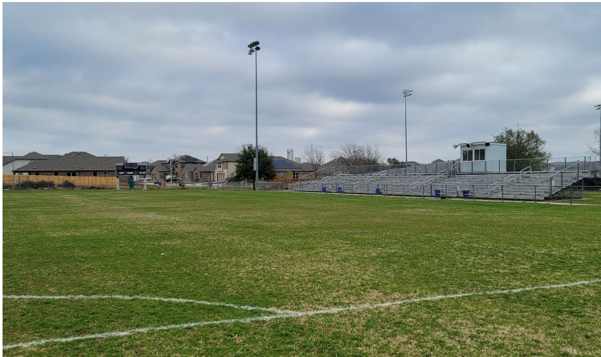
Football field lawn requires maintenance, and the site faces drainage issues. Artificial turf is desired.
