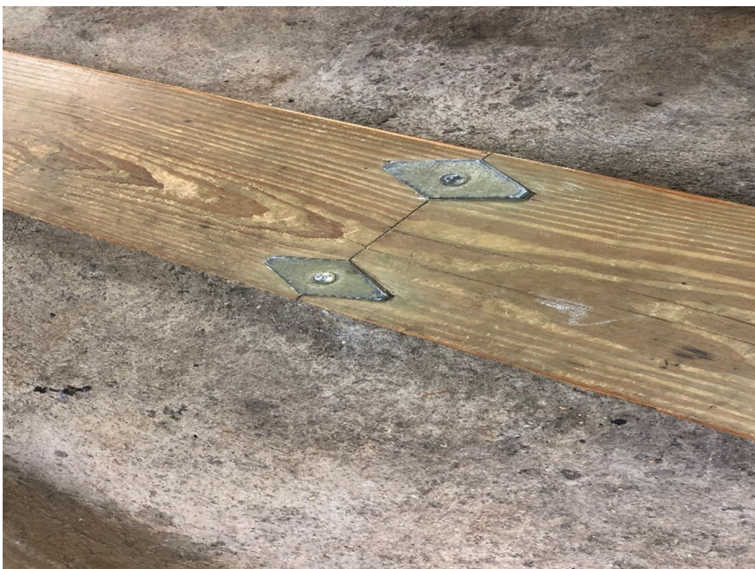
Rough connection between sections of bench seating for spectators.
