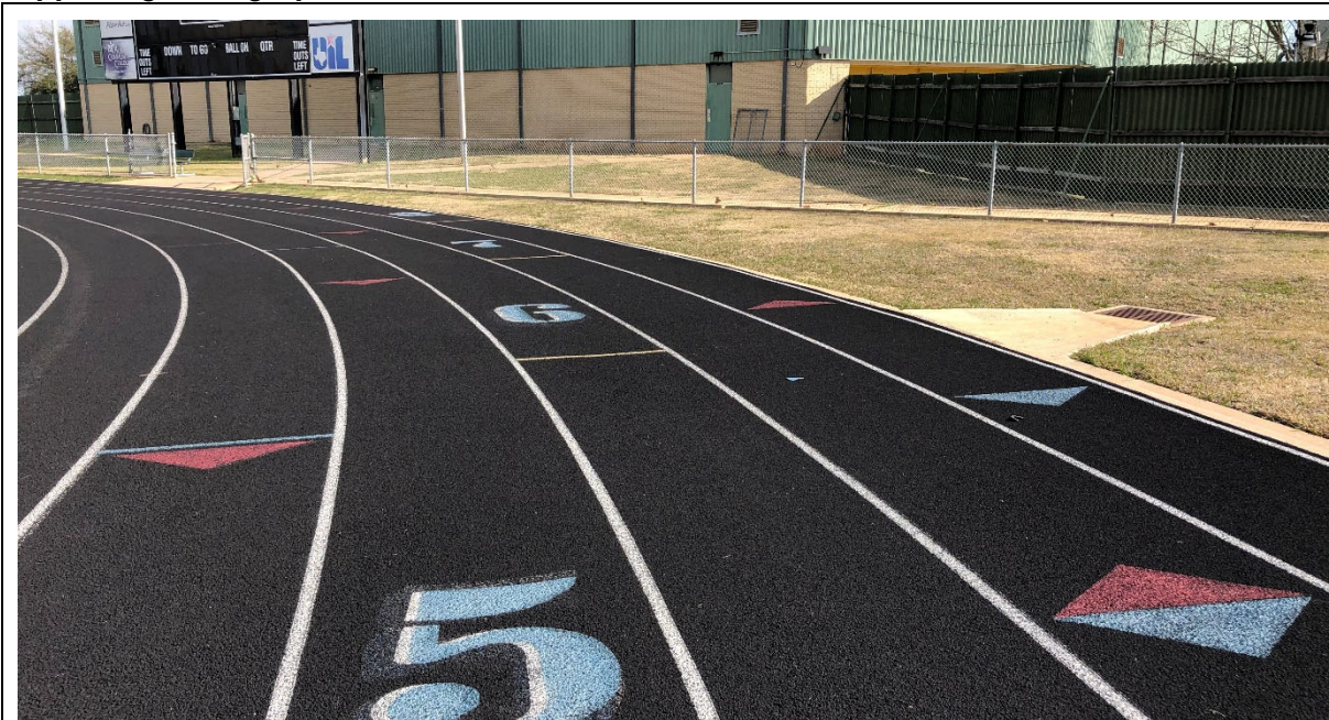
Track and scoreboard appear in good condition.
