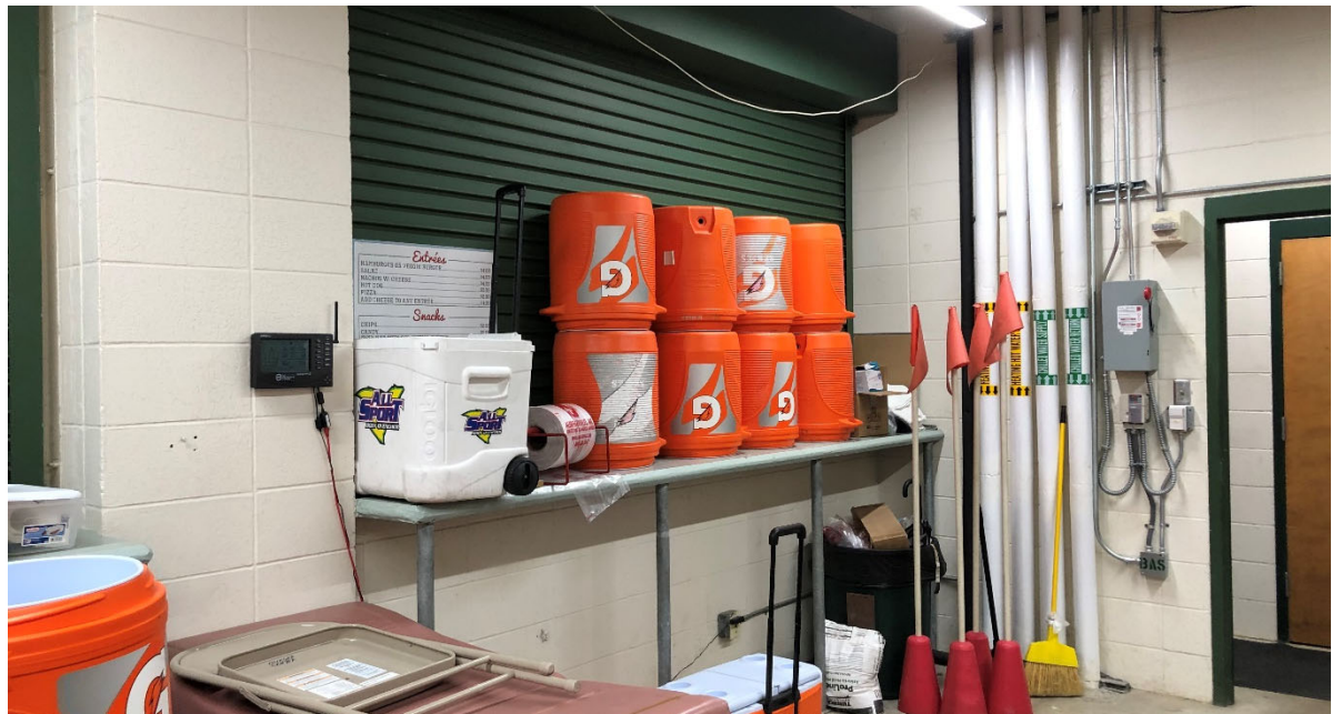
Exposed utility lines in the concession room.
