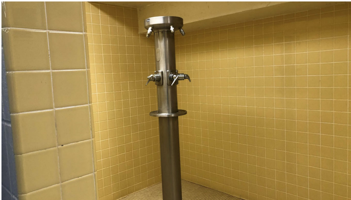
Shower area in locker/dressing room appears in fair condition.
