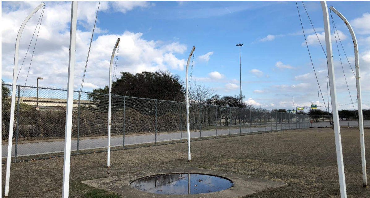
Discus cage frame appears in poor condition and rusted.
