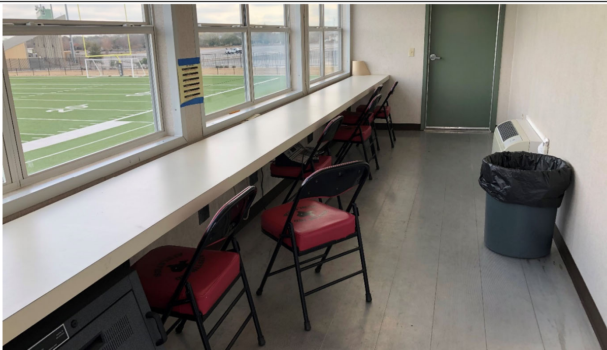
Press box of auxiliary field in good condition.
