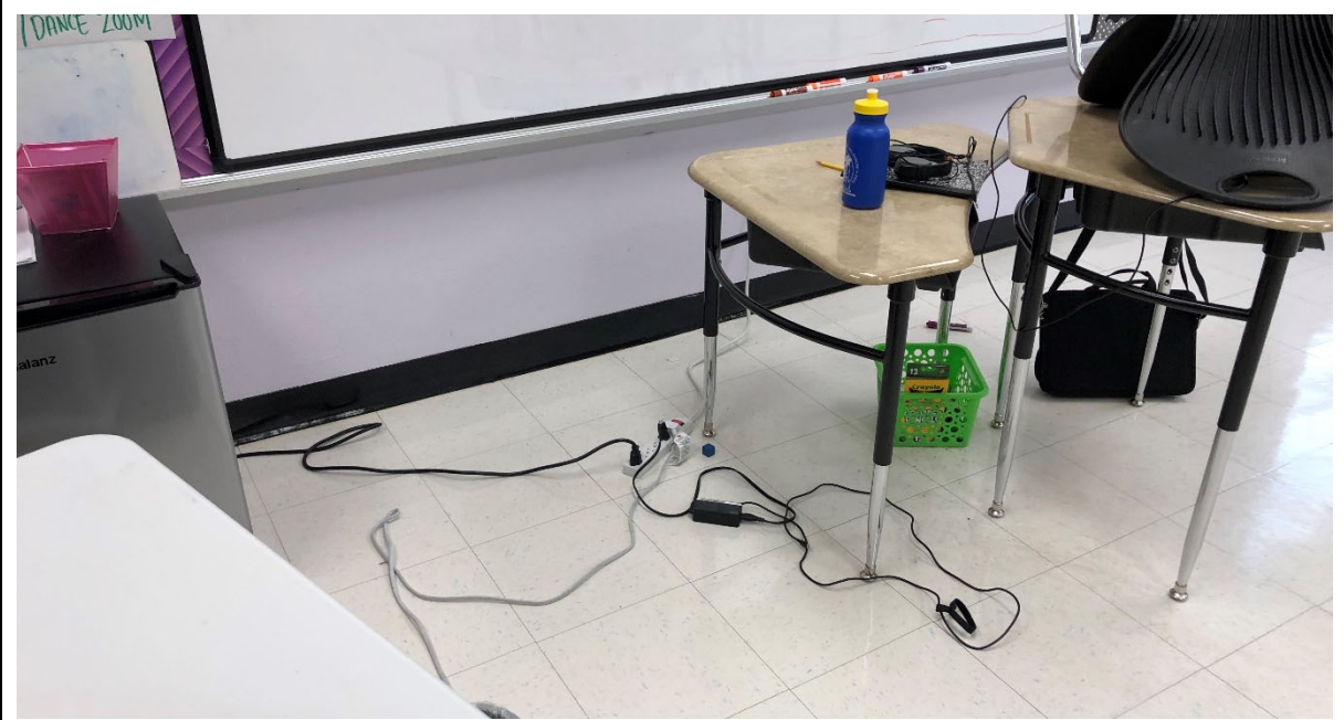
Typical studio device connections include extension cords and power strips.
