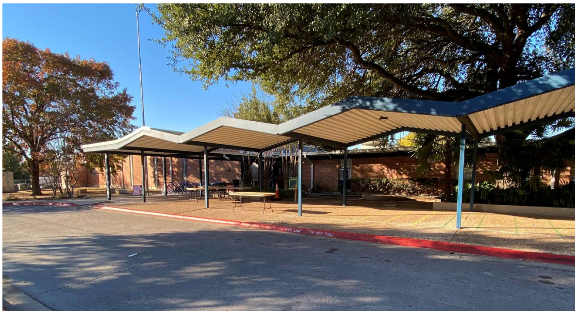
Blanton ES main entrance: Canopy also connects to door just out of view with inadequate signage to distinguish the main entrance.
