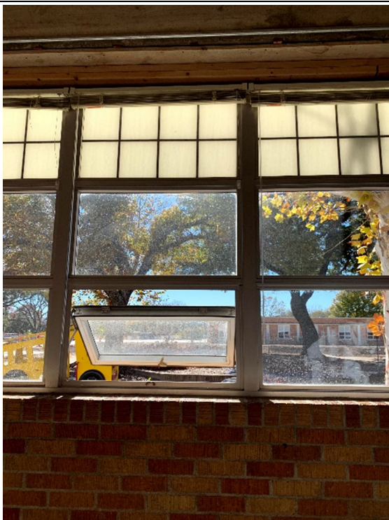
Interior: Existing windows to be replaced
