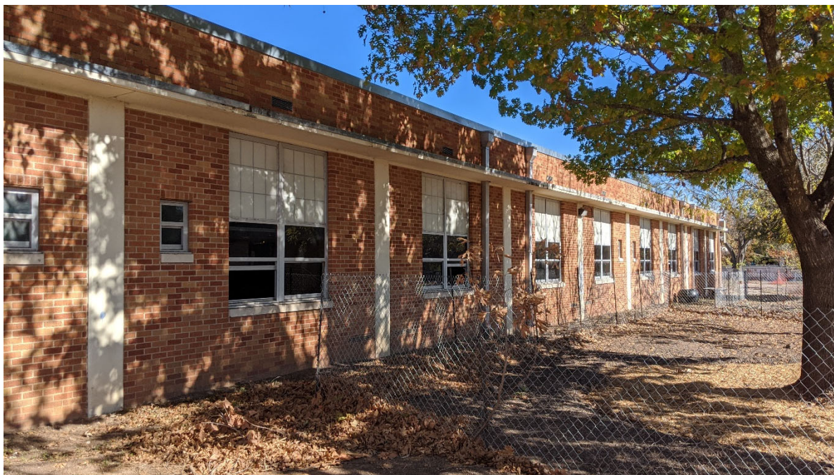
Exterior: Existing south wing south elevation.
