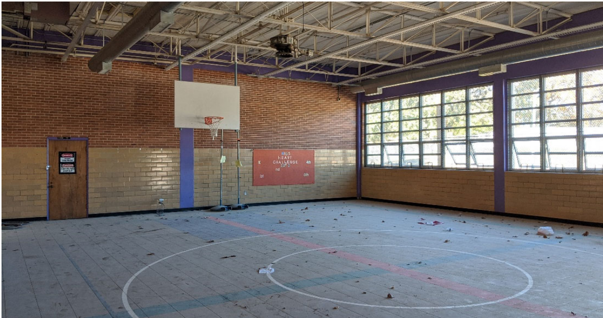
Interior: Existing gymnasium. To be replaced with new maker space.
