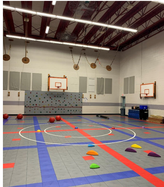
PE and Wellness: The gym connects to the cafeteria with an operable wall. The space is in good condition but aged.
