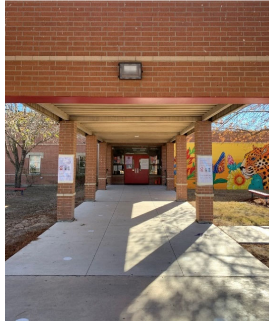
Front Entry: Main entrance is difficult to identify when approaching the building. Added wayfinding or signage could improve visibility.
