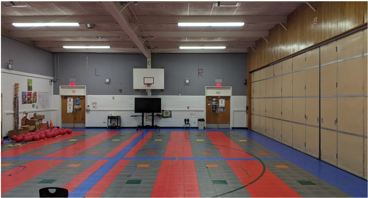
PE and Wellness: Gymnasium area is undersized per Ed Spec and has a movable partition to the cafeteria.
