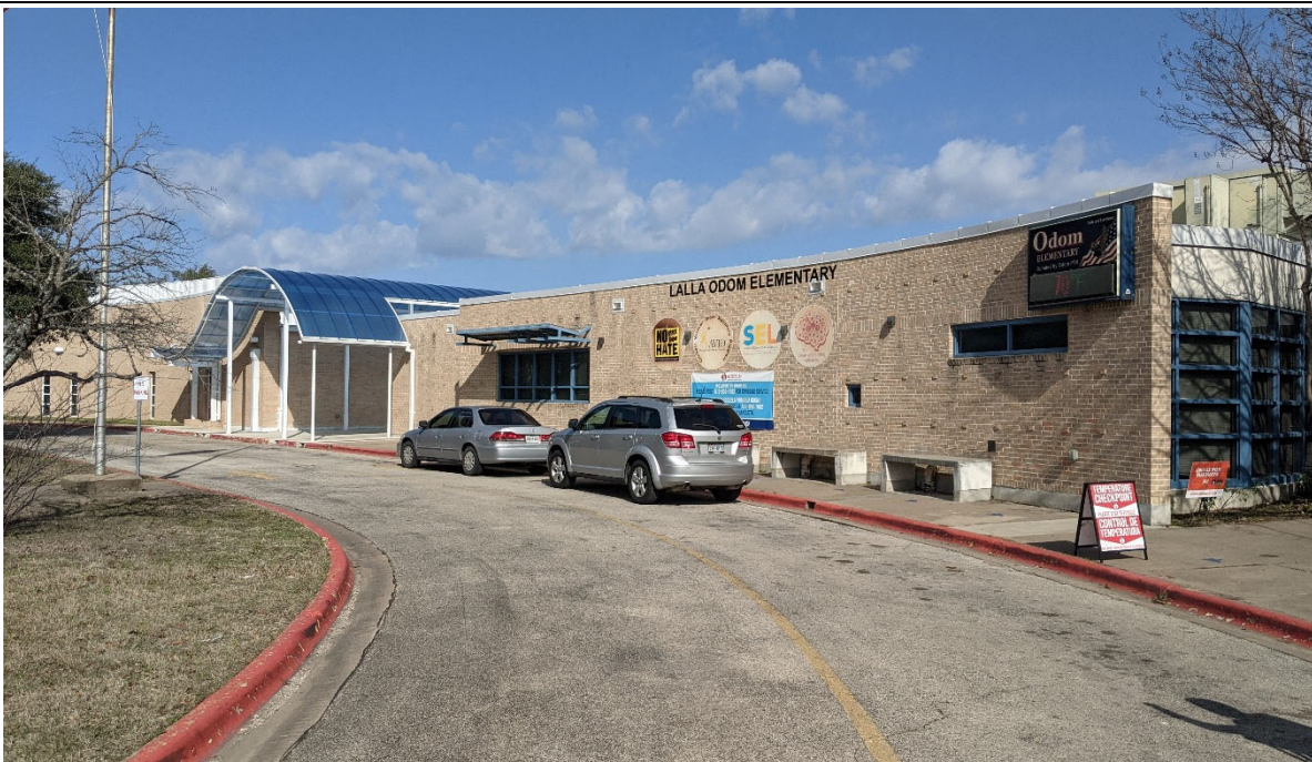
Exterior: Main entrance with new curved canopy.
