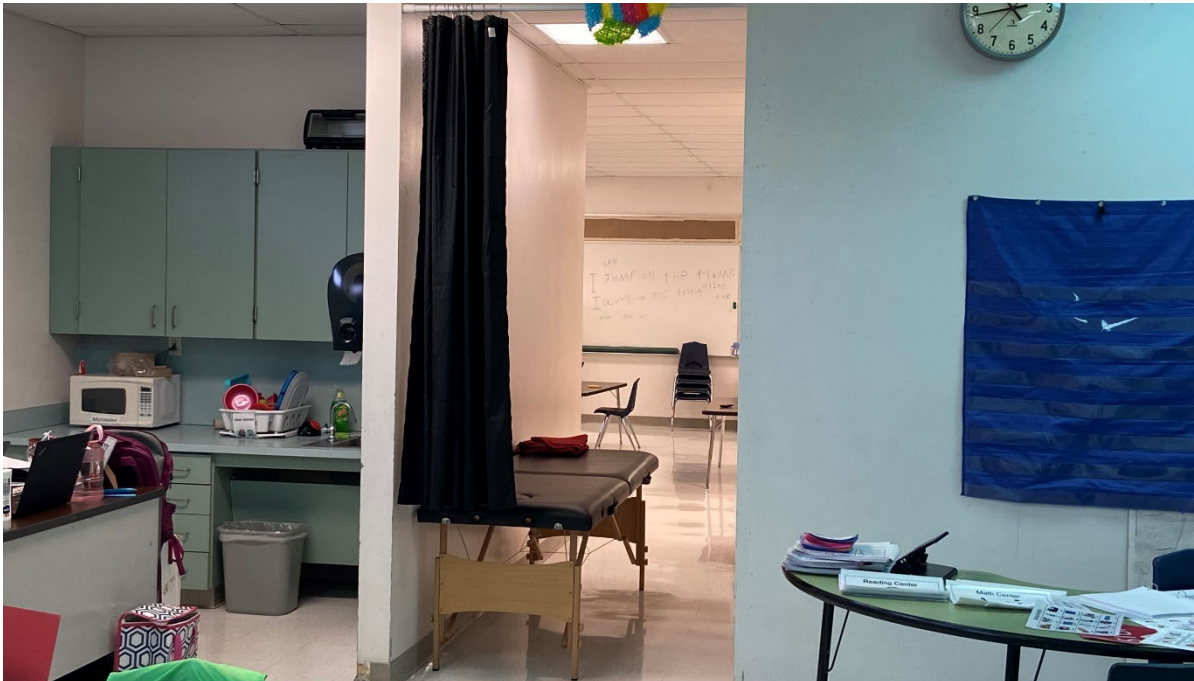
Restroom corridor at special education room with changing table unable to fit in restroom. Placement of a curtain provides inadequate privacy.
