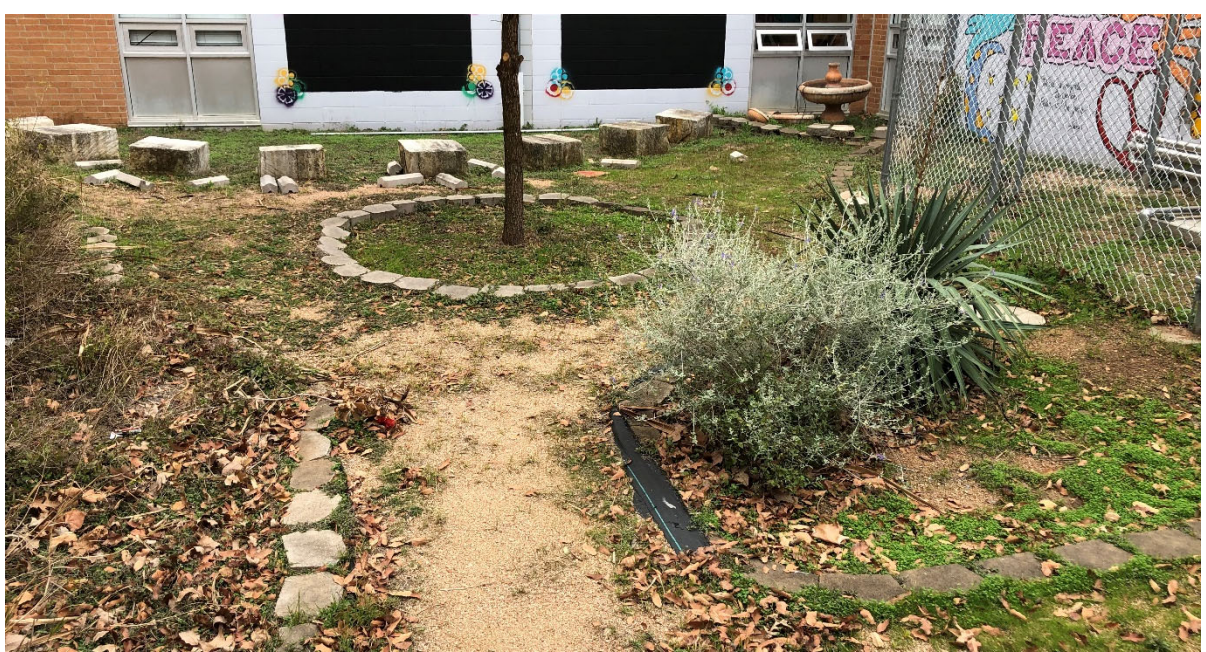
Small courtyard space between studio wings is used as an outdoor learning area but does not have direct access to the building. Space is fenced in and lacks a developed walkway for access, and therefore is not ADA accessible.
