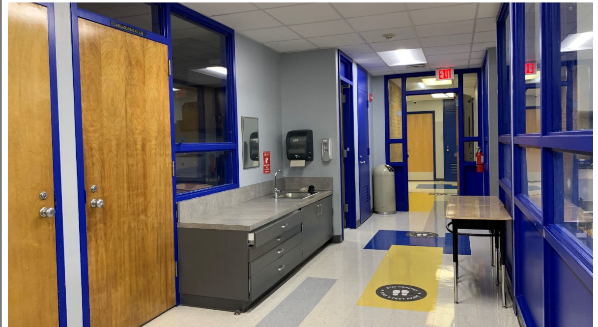
Renovated Studio Corridor: The studios have great visibility to the corridors; however, the quality/thickness of glass compromise acoustics.
