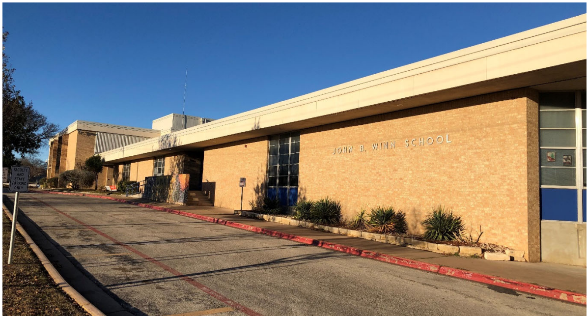
The main entry is difficult to locate. Wayfinding could be improved. There is no canopy.
