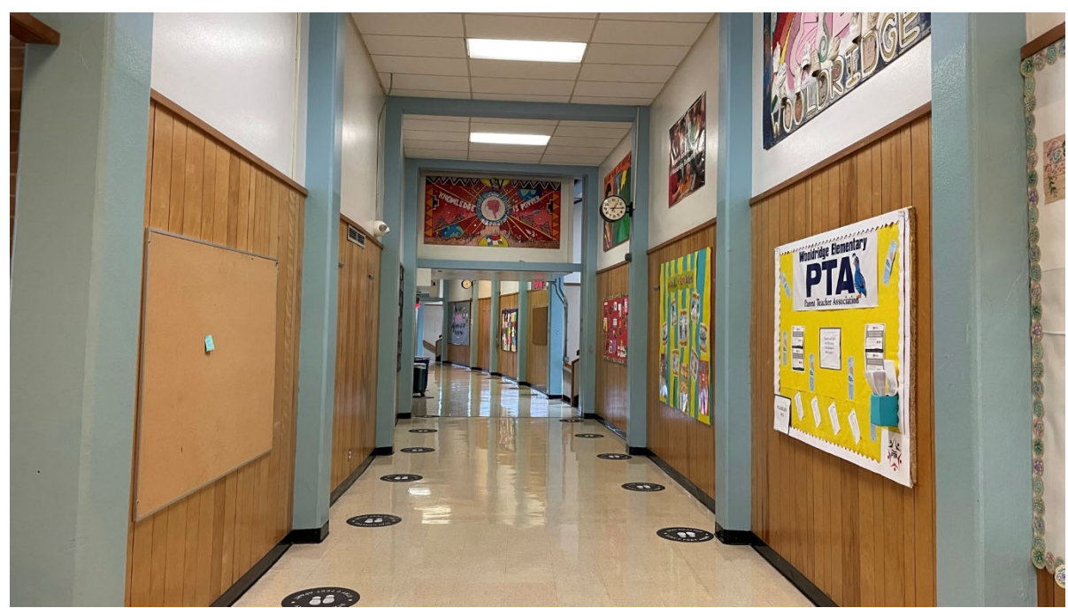
Corridor (Main Building): Corridors lack transparency, collaboration areas or display. There is very little natural light.
