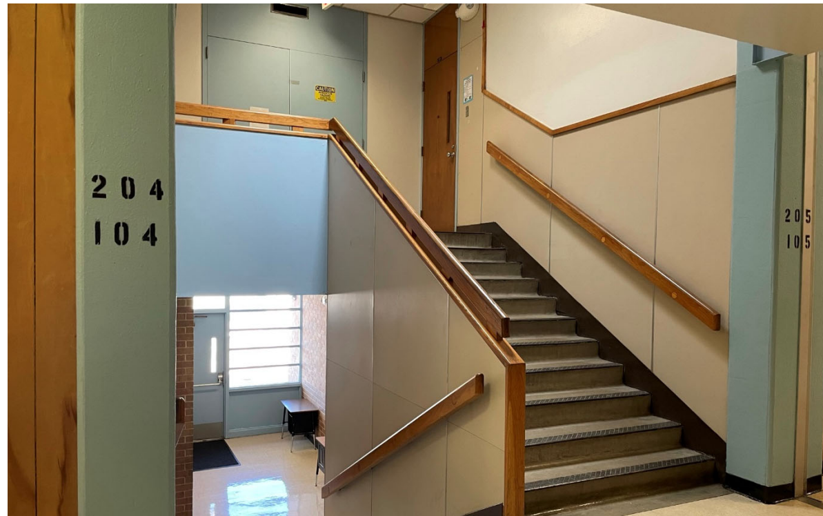
Corridors (Main Building): Studios can only be accessed from main corridor by going up or down a flight of stairs. A ramp and lift are provided at either end of the building
