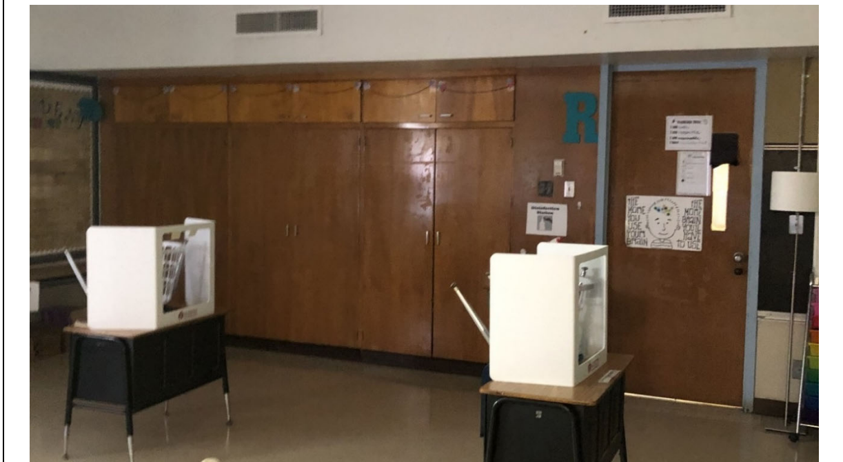
Typical Studio (Main Building): Each studio has existing built-in storage that is underutilized and discourages flexibility. There is no visibility into corridors.
