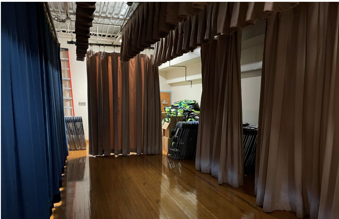
Visual and Performing Arts: Stage is not accessible and lacks storage.
