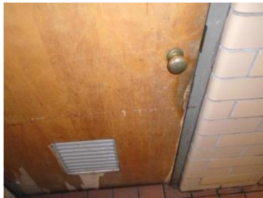
Interior wood door at end of life
