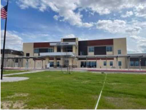
North Elevation, Main Entrance
