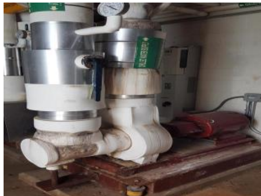
Corroding pipe
