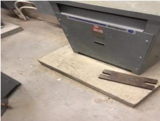
Exposed base of unit
