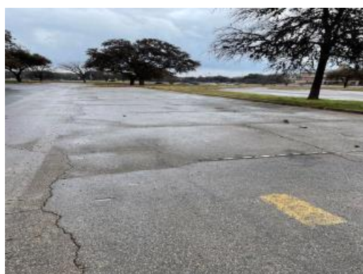
Cracked asphalt
