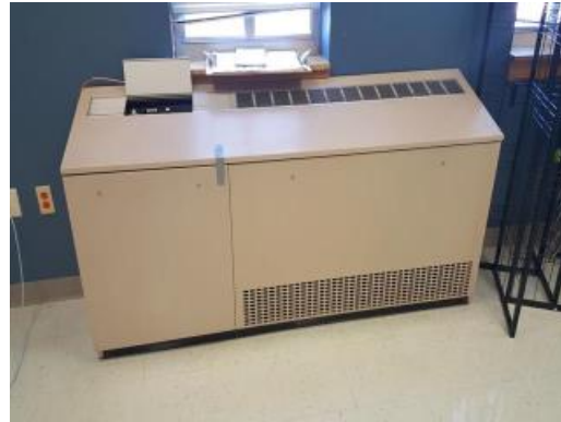
Ground Source Water Source Heat Pump
