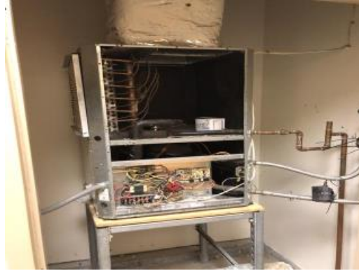
Exposed wiring
