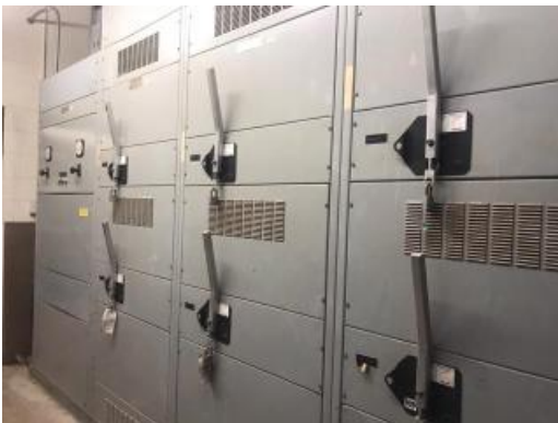
Switch gear past useful life
