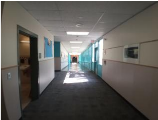
Main building hallway
