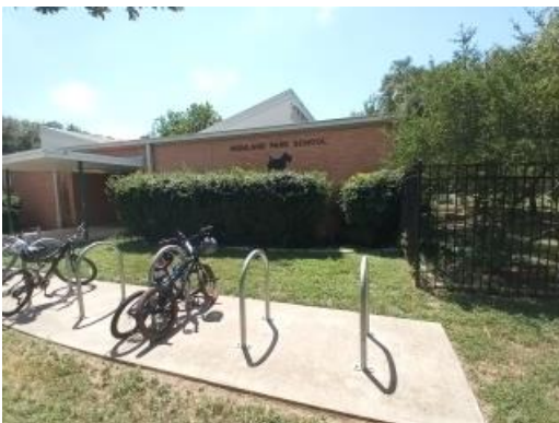
External bike racks
