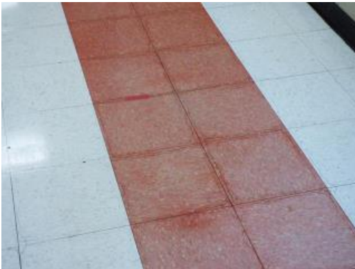
Vinyl composite tile (VCT) well worn
