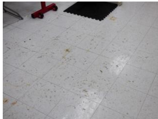
Vinyl composite tile (VCT) is worn
