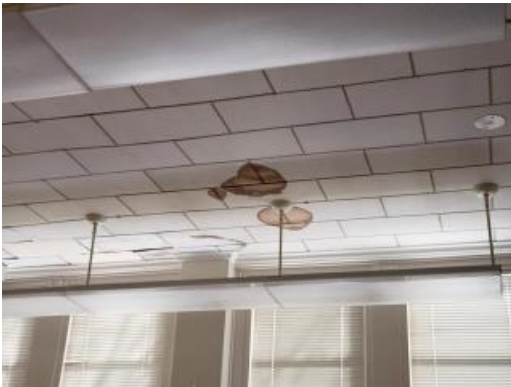
Stained concrete masonry unit
