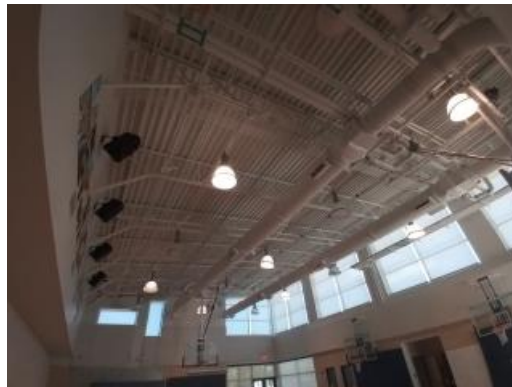
Gymnasium roof structure
