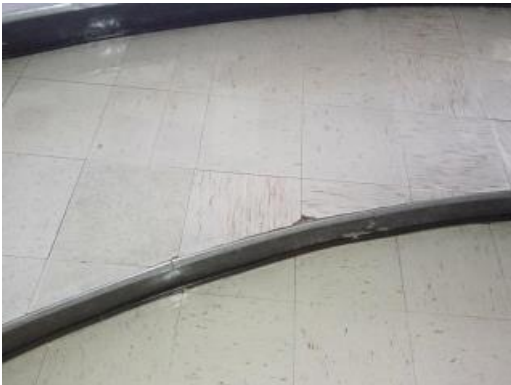
Worn vinyl composition tile flooring
