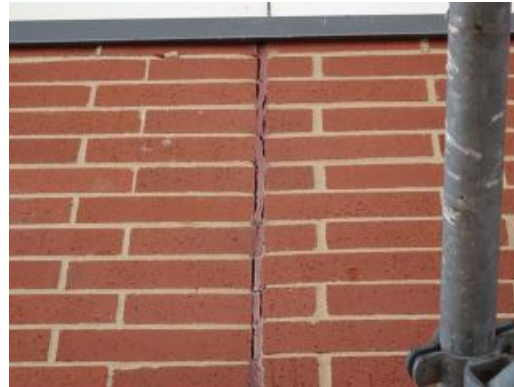
Brick Control Joint
