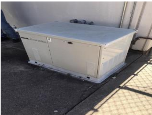
Rooftop electrical system
