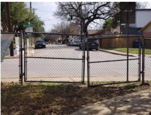
Warped/damaged gate
